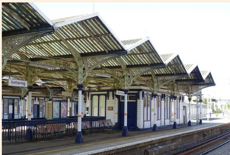
Kettering Train Station
