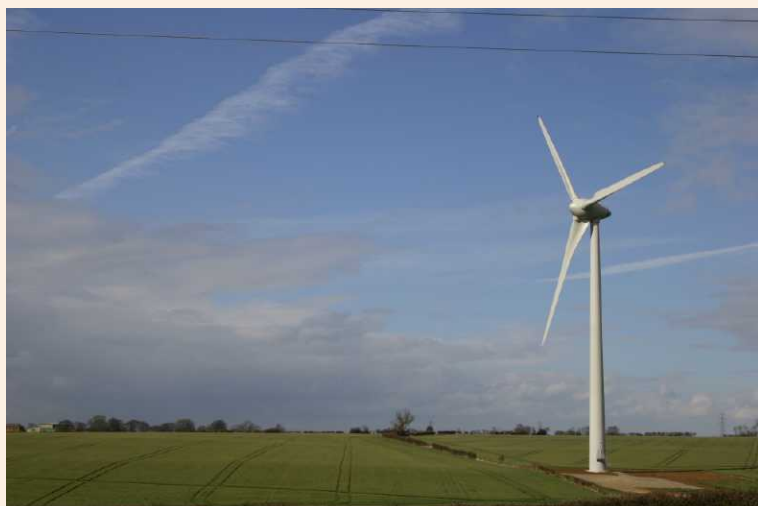
Wind Turbine at Burton Wold Wind Farm
